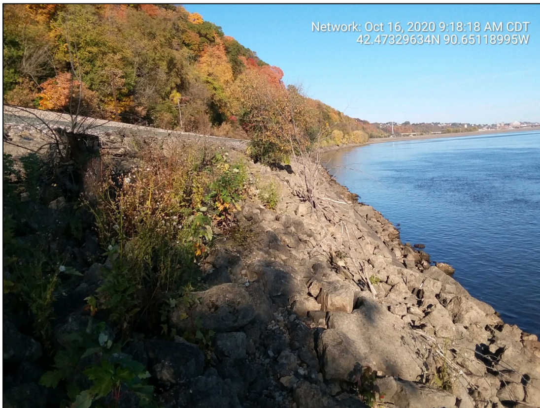
Figure D-2: Typical Photograph of Project Site
